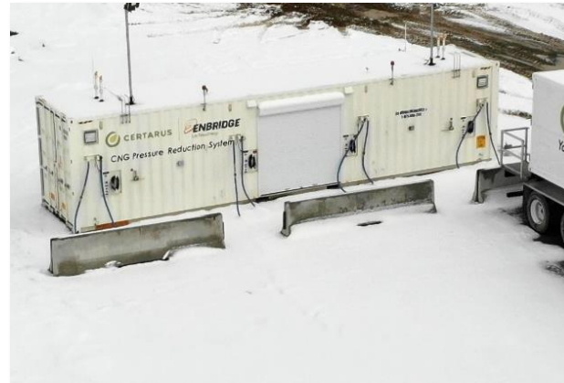
Modular CNG/RNG/Hydrogen Pressure Reduction Systems – Containerized pressure reduction systems for long-term deployment to customer delivery locations
