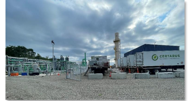
Juniper Ridge - Maine Landfill: Project recently came online delivering 2-3 loads daily
